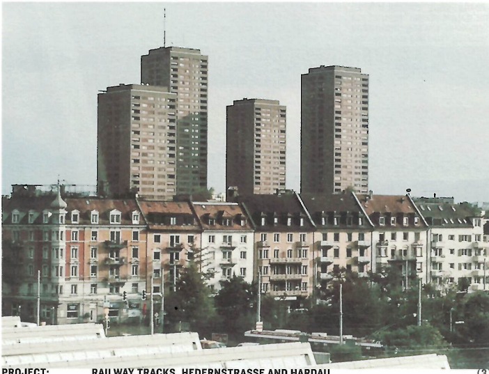
PROJECT: RAILWAY TRACKS, HEDERNSTRASSE AND HARDAU (3) LOCATION: ZÜRICH (ZH) IMAGE: PHILIPPE JORISCH
