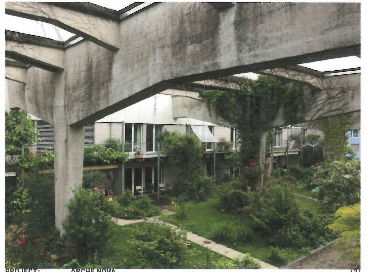
PROJECT: ARCHE NOVA (2) ARCHITECT: SUTER+SUTER LOCATION & YEAR: USTER (ZH), 1991 IMAGE: JOM ARCHITEKTEN
